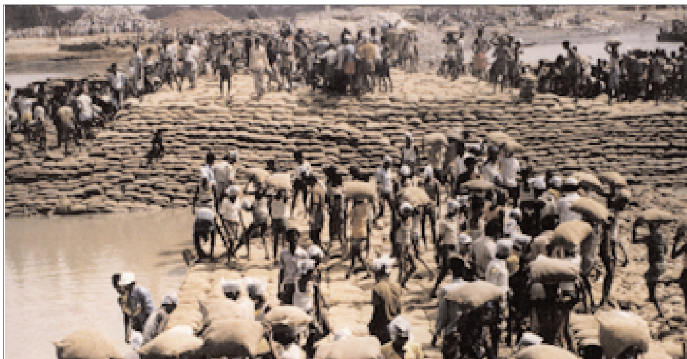
The closure of a tidal inlet by a multi purpose dam (irrigation, flood protection, communication and land reclamation) by the men power of 5000 people during one tidal cycle.
