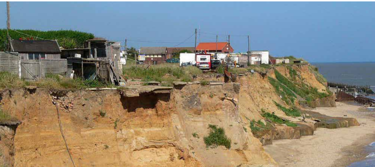
Severe cliff erosion threatening the coastal settlement of Happisburgh, UK. (photo: EUROSION)
