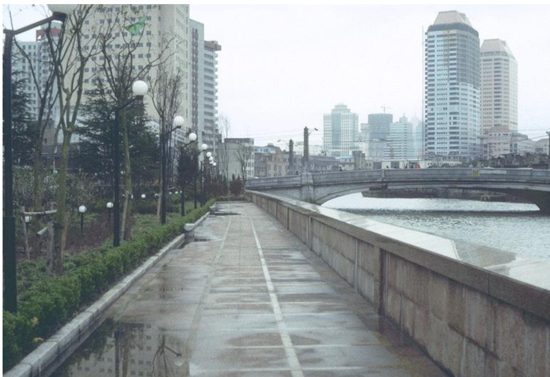
Renewal of Suzhou Creek embankment and flood wall. (photo: Peter Kerssens)
