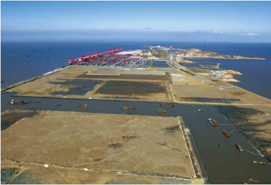
Figure 6: Donghai Cross-sea Bridge (in the horizon) and Yangshan Harbour The project started in June of 2002 with the construction of the 32.5 km long Donghai Cross-sea Bridge connecting Shanghai and Yangshan Harbour; the opening of Yangshan Harbour: December, 2005; the Phase-3 of Yangshan Harbour finished in December 2008. The Yangshan Harbour key reached a length of 5600m. The whole project will be finished in 2020. (source: http://en.wikipedia.org/wiki/File:Yangshan_Deepwater_Port.jpg )
