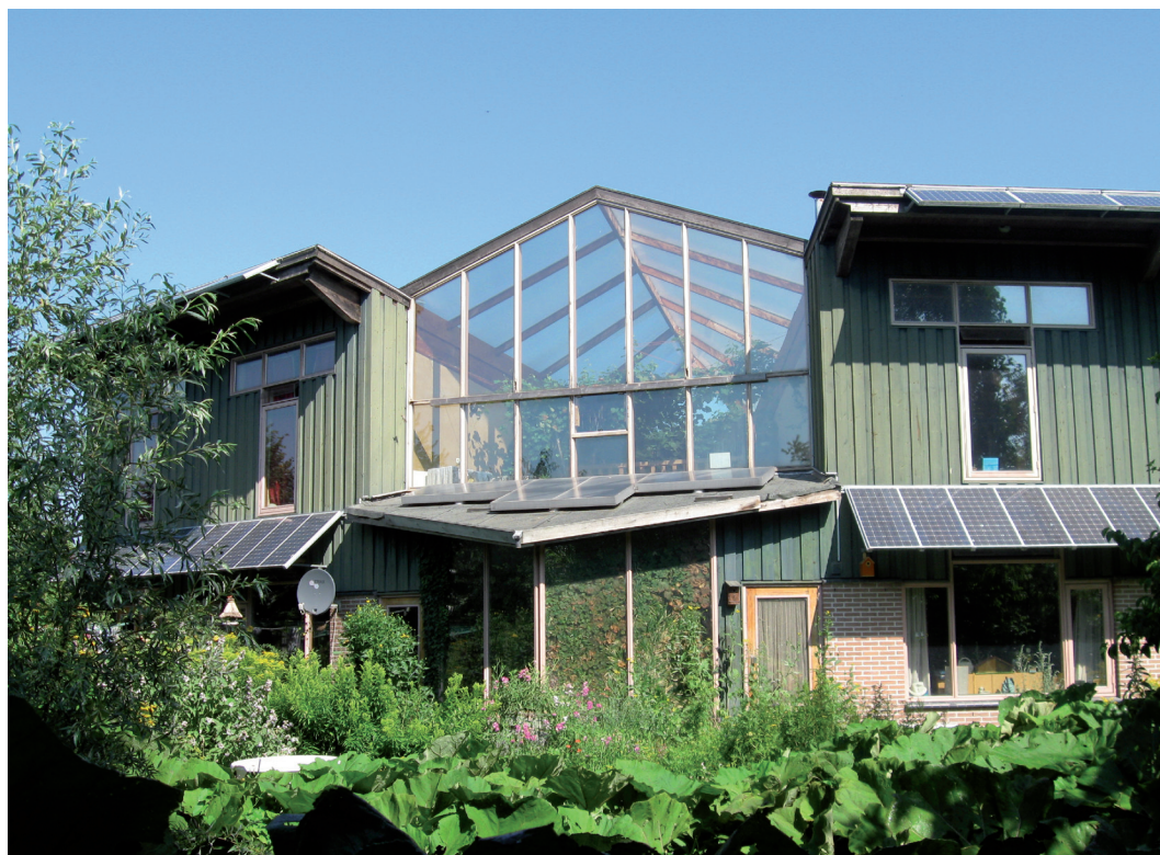
Our ECOHOUSE & ECOSAVE Office, Flevoland, Holland, trapping the solar radiation in the central greenhouse part of the building, with solar PV and thermal panels and rain water collection and waste water purification in the garden. (photo: D. Vandy)
